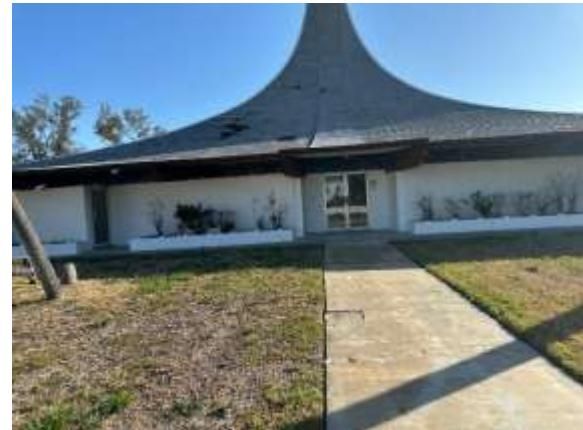
Roof: The subject has a architectural roof with a asphalt shingle surface. There are gutters and leaders to provide water drainage away from the roof surfaces. Areas of the roof needs repairs due to recent hurricanes.
