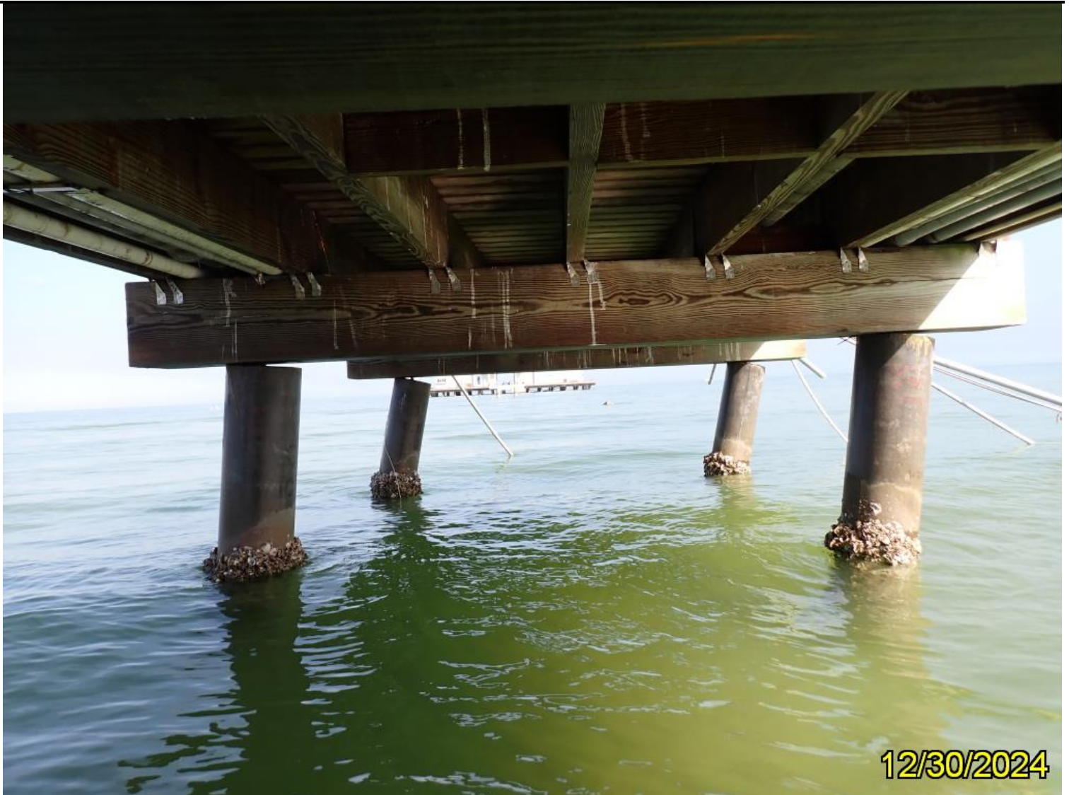
Photo 12: Element 227 Re Conc Pile
