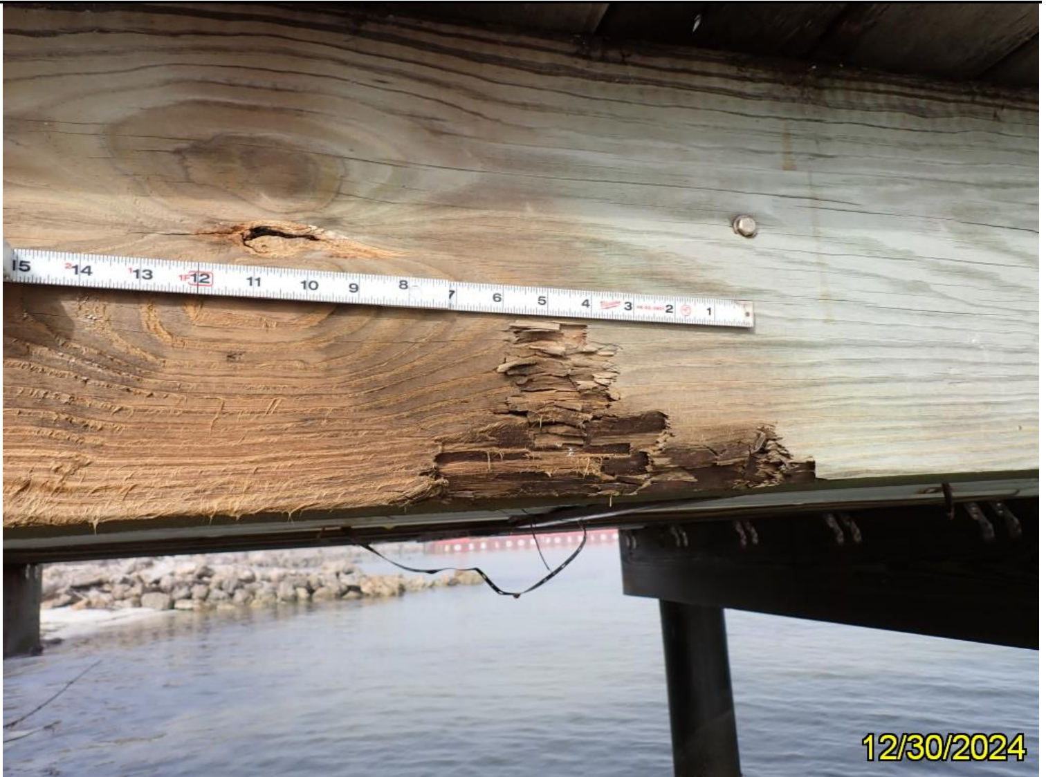
Photo 20: Element 111 Timber Open Girder
