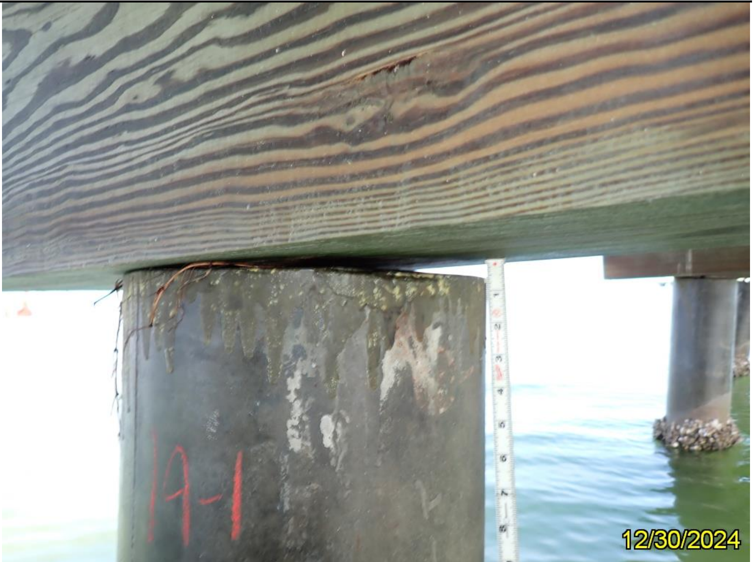
Photo 10: Element 227 Re Conc Pile
