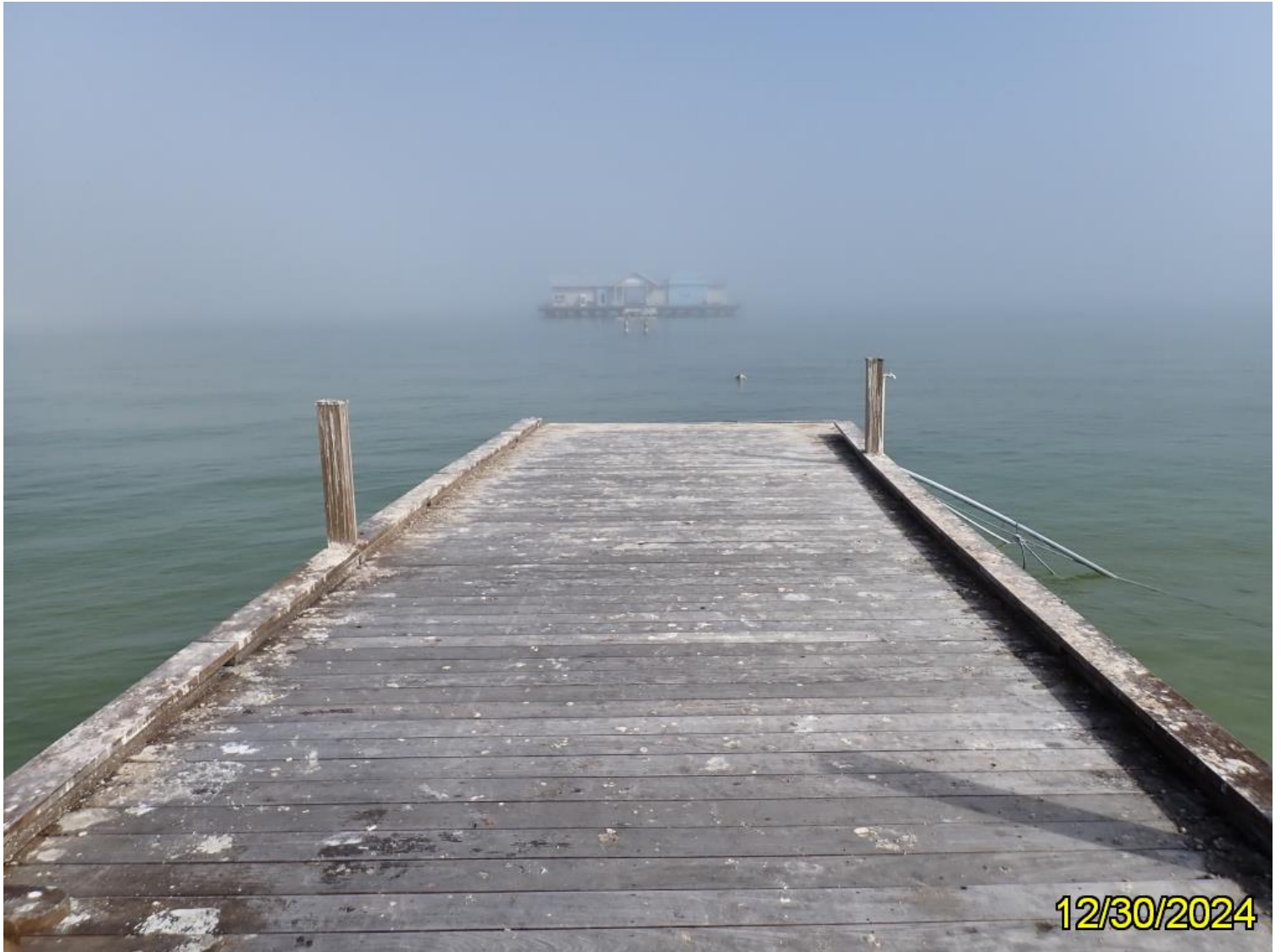
Photo 1: Elements 60 Other Deck & 227 Re Conc Pile & 235 Timber Pier Cap & 111 Timber Open Girder
