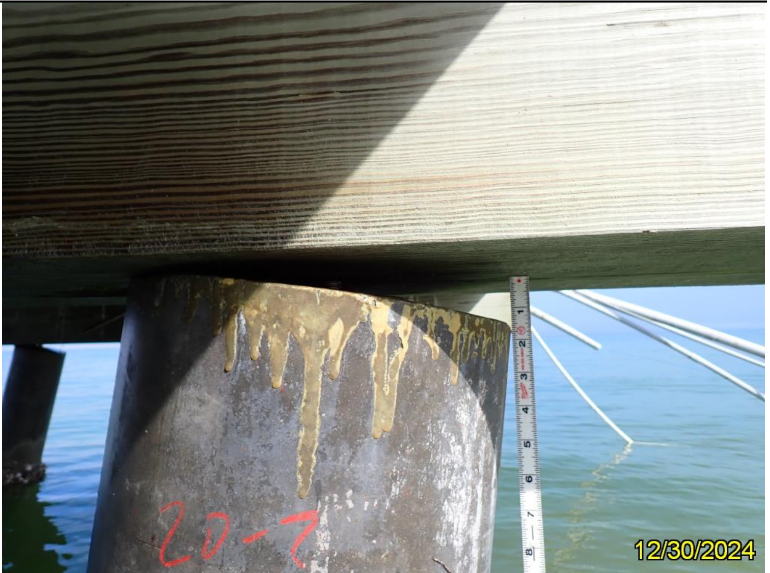
Photo 14: Element 227 Re Conc Pile
