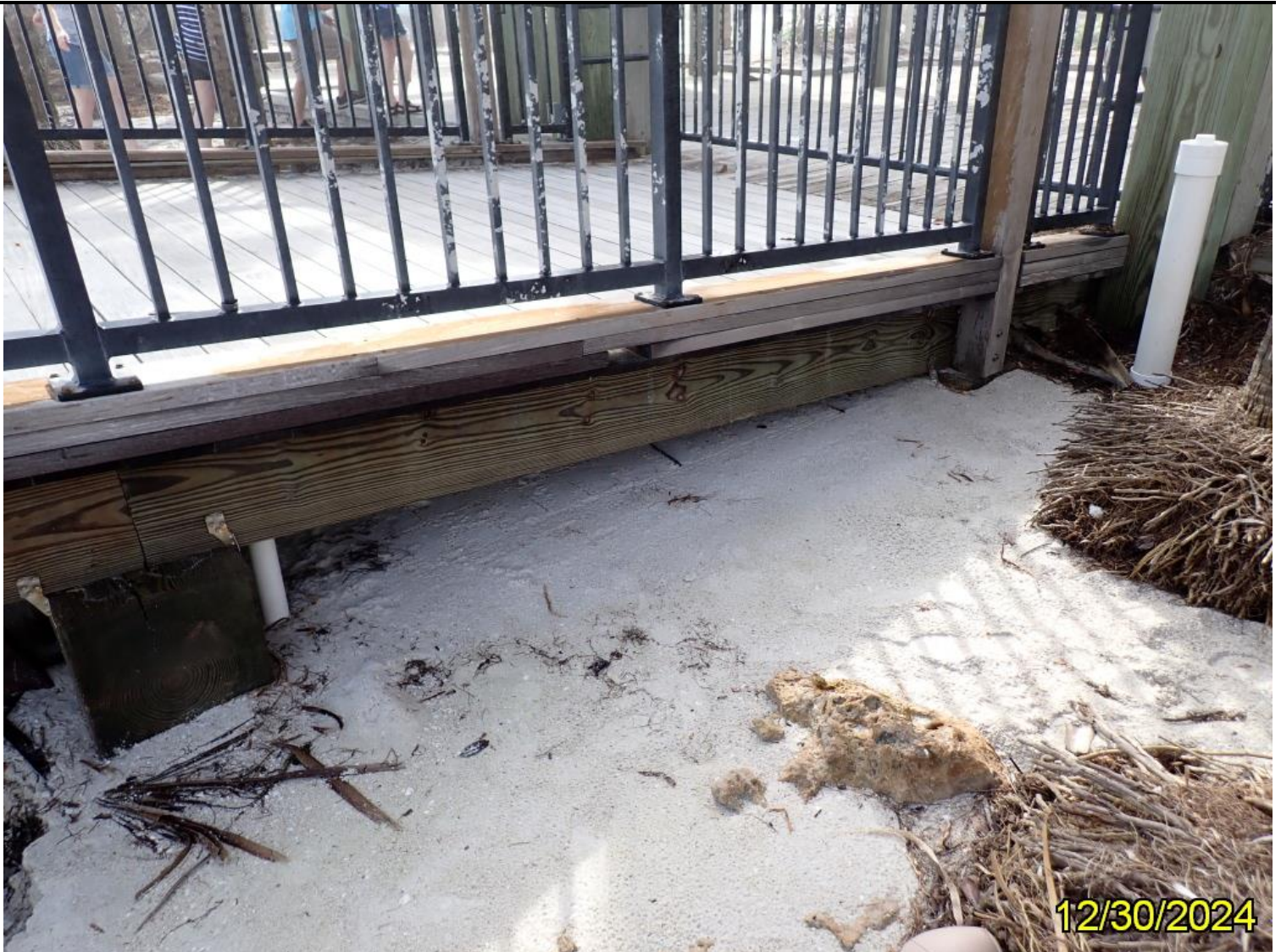
Photo 8: Element 216 Timber Abutment
